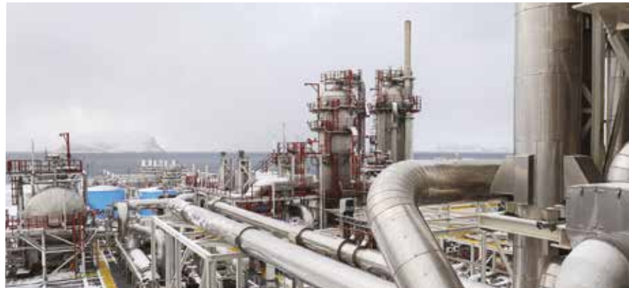
Melkøya LNG plant with CO 2 separation. Photo: Statoil/Helge Hansen
